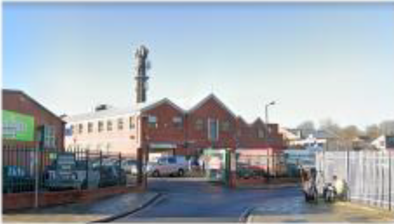
Existing buildings view from Wells Way
