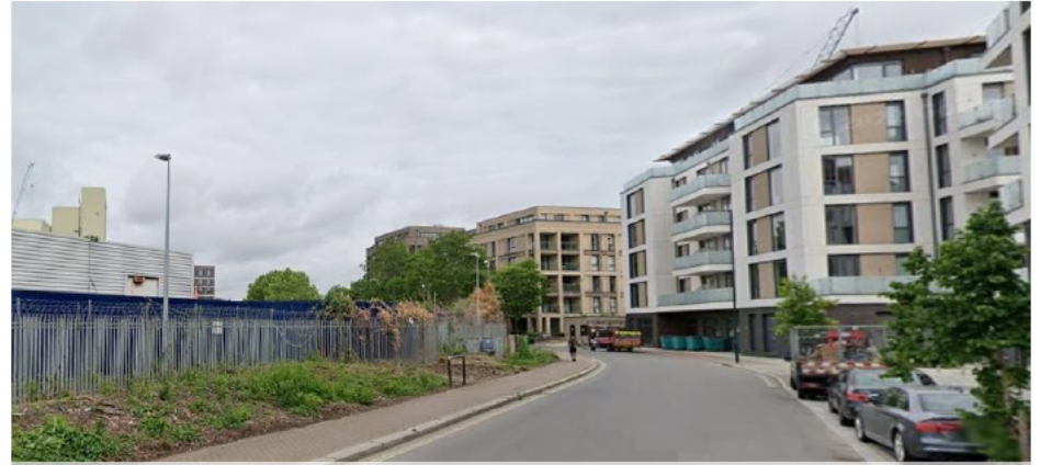
View north from outside Quebec Quarter
